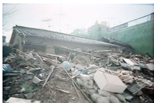
Collapsed Residential Structure
